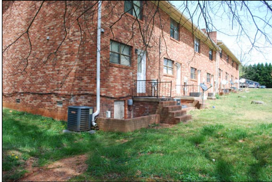
Photograph 1. Modern Apartment Buildings Adjacent to the Dysart-Martin House to the East
