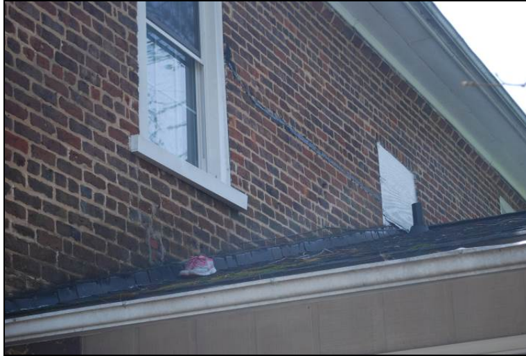
Photograph 12. Second Floor Window Partially Concealed by Rear Addition
