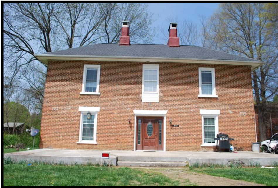
Photograph 5. Dysart-Martin House, Façade (South)
