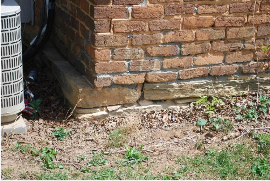
Photograph 6. The continuous Rough-Cut Stone Foundation
